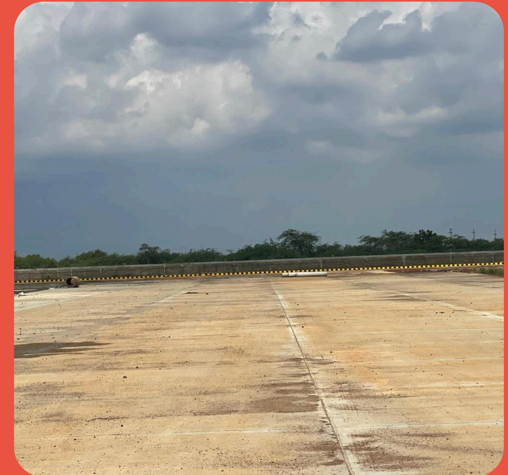
**AN INLAND CONTAINER DEPOT (ICD) WITH 275METERS LENGTH \* 30 METERS WIDTH HAS BEEN DEVELOPED WITH IN THE FTWZ PREMISES TO FACILITATE EFFICIENCY HANDLING , STORAGE, AND MOVEMENT OF IMPORT AND EXPORT CONTAINERS.**
